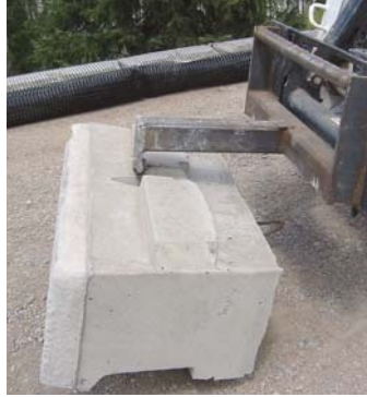
A block being set in place with a skid steer.
